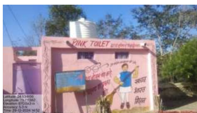
Figure 43: Toilets built by HDFC in Kag Madarda school
