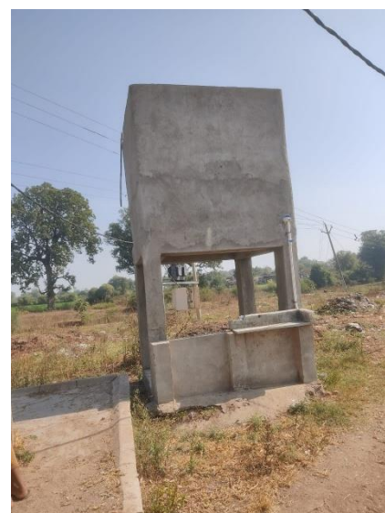
Figure 3 Half constructed Jal Minar (Water tank) in Rampur Kalan
