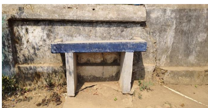
7 Incomplete structure without pipe connection from water tank in Toyimuda Middle School
