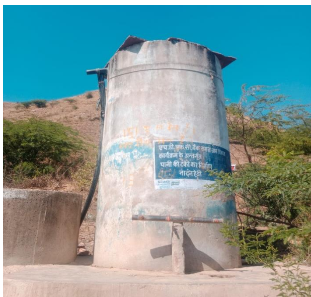
Figure 26: Water Tank- H&H
