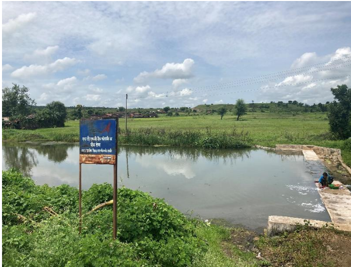
Image 2: Check Dam built under HRDP in Rajdongri Village, Madhya Pradesh
