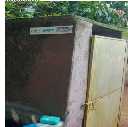
Image 4: Sanitation infrastructure built under HRDP in Hatnabeda, Jharkhand
