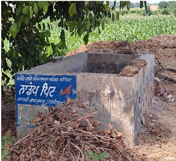
Image 2: Water infrastructure built under HRDP in Punjab
