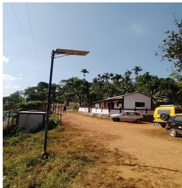
Image 7: Solar Street Light installed in Pahamshken village
