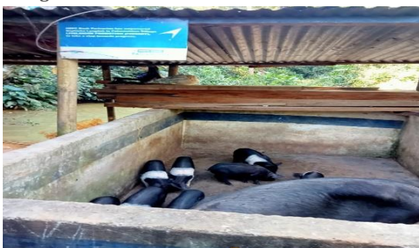
Image 8: Pig pen constructed in Pahamshken village
