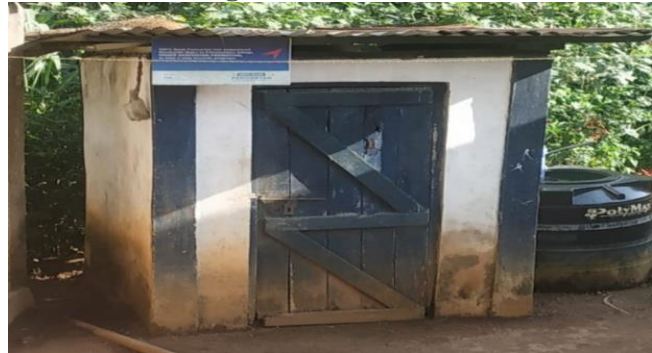
Image 13: Household Toilet constructed in Pahamshken village
