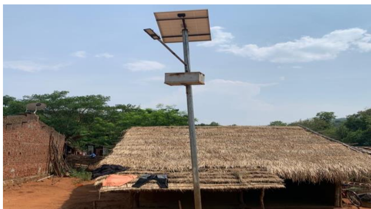
Figure 12: A Solar Light Installed in a Project Village
