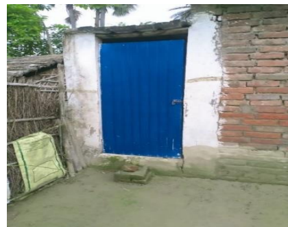
Image 8: Sanitation infrastructure built under HRDP in Bihar
