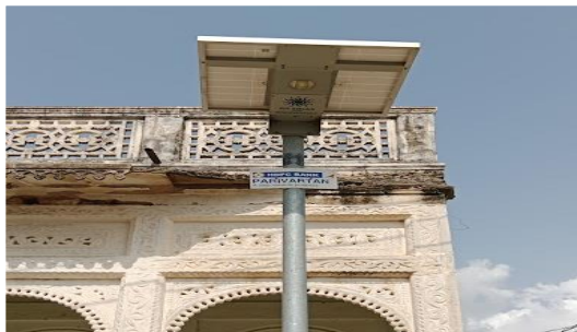
Figure 12: A Solar Light Installed in Bayal
