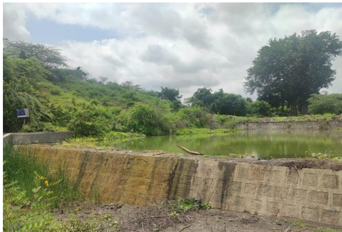
Image SEQ Image \* ARABIC 1: Check dam built under HRDP in Khamtane village, Nashik
