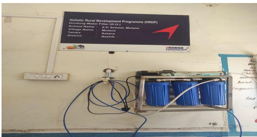
Image SEQ Image \* ARABIC 11: Installation of RO Filter, Mulane, Nashik
