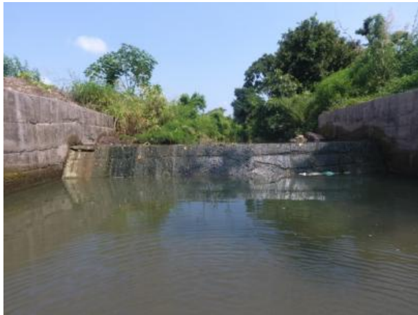
Image 1 Check dam construction, Yevti village, Washim
