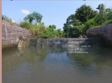
Image 3 Check dam, Yevti village, Washim
