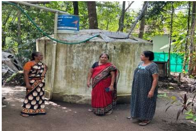
Image 2: Rainwater harvesting unit in Alappuzha (10,000 Litre capacity)
