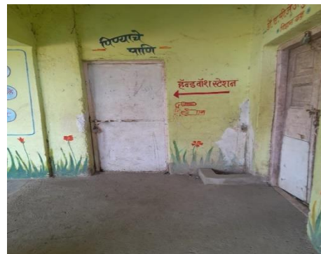
Image 10: Hand wash station, Puyni
