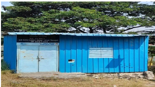
Image 9: Installation of RO filter, Puyini village, Nanded
