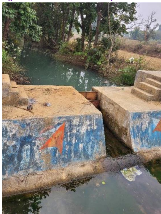
Figure 13: Check-dam in Rukhpur
