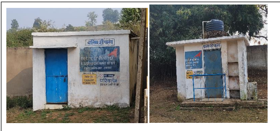
Figure 37: Separate washrooms for boys and girls in a school in Ramnagar
