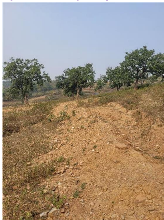
Figure 13: Trenching in Ranpur
