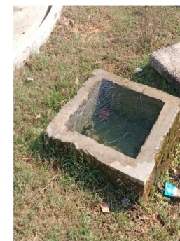
Soak Pit in the project area
