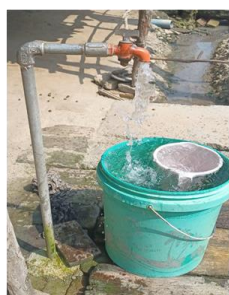
Water tap installed at Banyani Village
