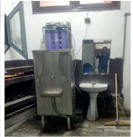
Water Structure repaired at GSSS Sahnewal
