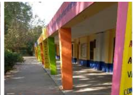
BaLA work on pillars at GSSS Sherpur Kalan
