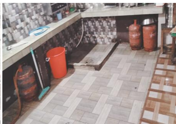
(f) Renovated MDM kitchen
