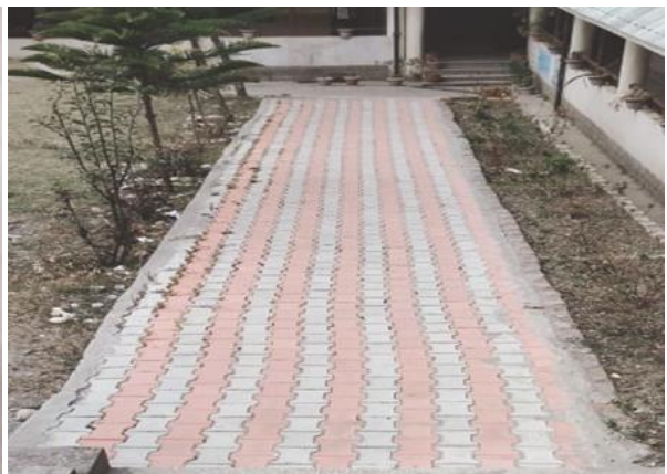
(j) Tiled pavement
