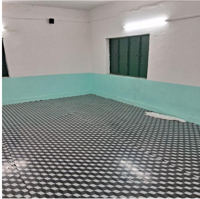
Image 1 Walls inside the classroom
